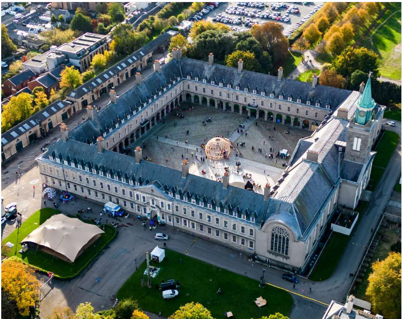
The 48-acre IMMA campus at the Royal Hospital Kilmainham
